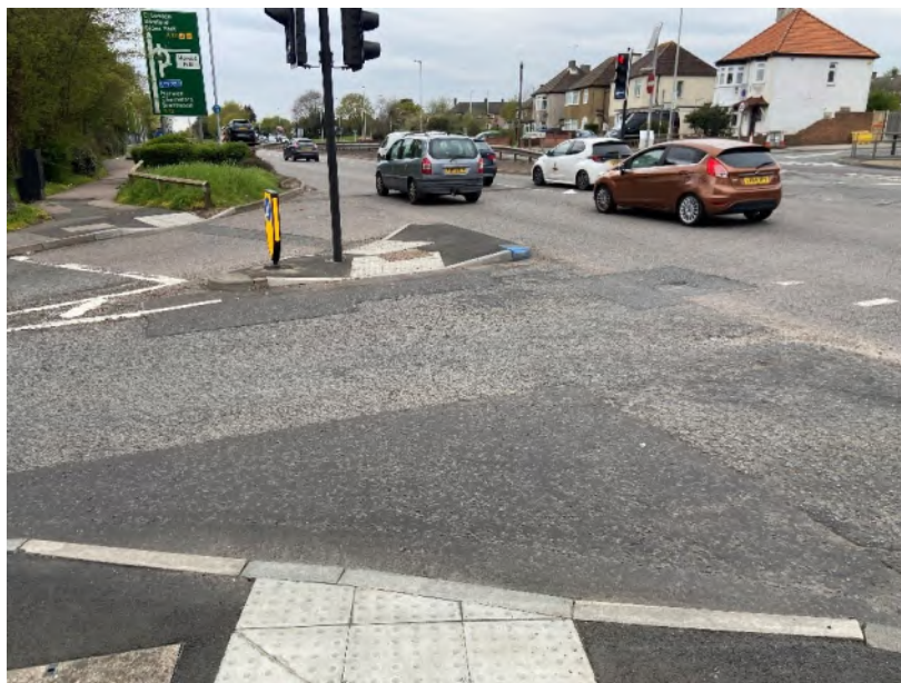
Photograph 4.1: Informal crossing facility on Harold Court Road
